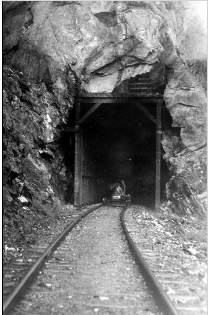
Figure 2.9. Leveling crew entering tunnel on velocipede. USC&GS Season’s Report Odessey 1923.
