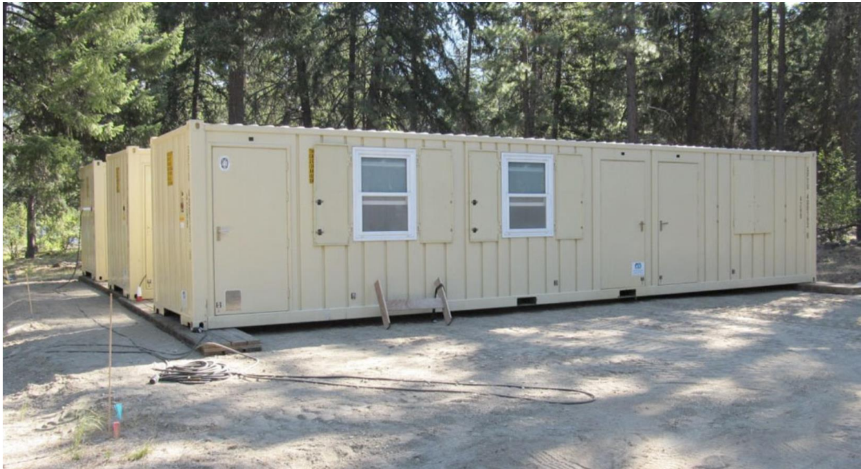
Personnel Camp at Lucerne for Holden Mine Remediation Workers.
