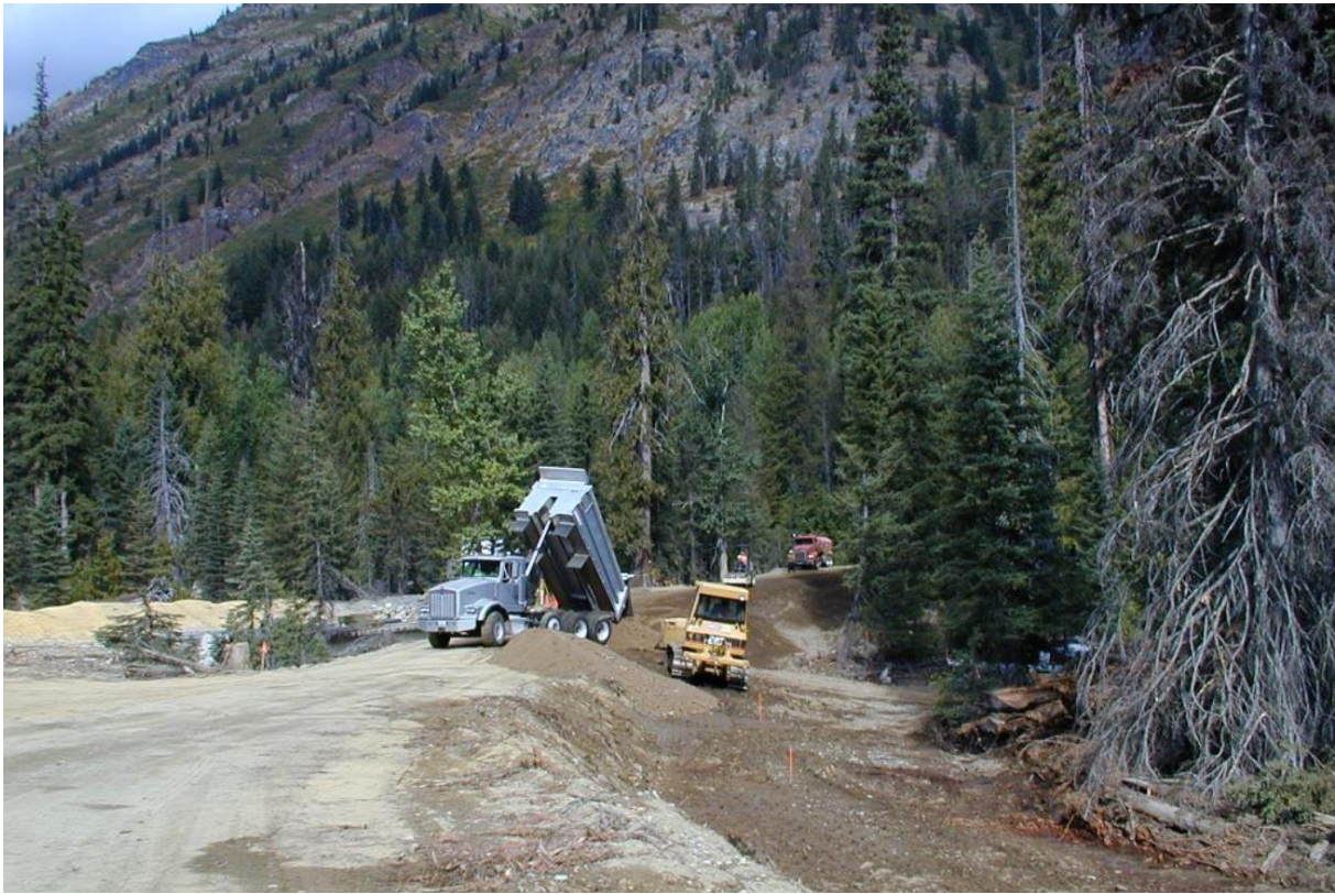
West bypass road construction, filling and grading the road surface.
