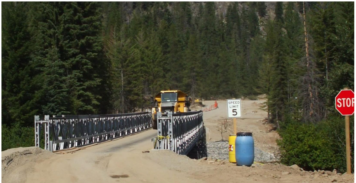
Bypass bridge over Railroad Creek completed and in use.
