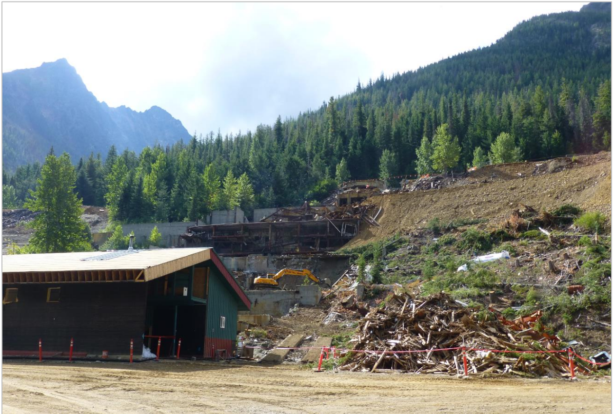
Holden Mill structure demolition.
