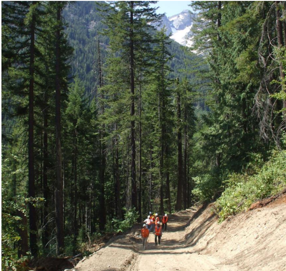
Rock quarry investigation pioneer road.
