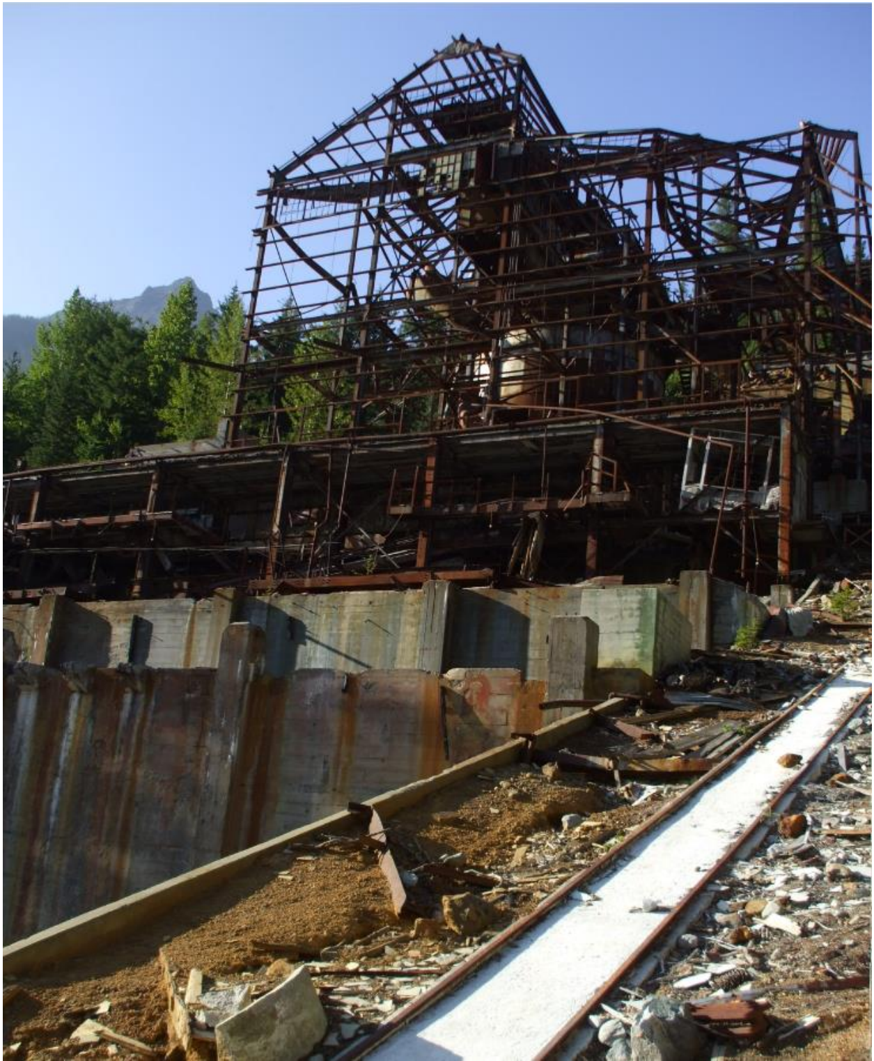
Holden Mine Site view of Mill Building
