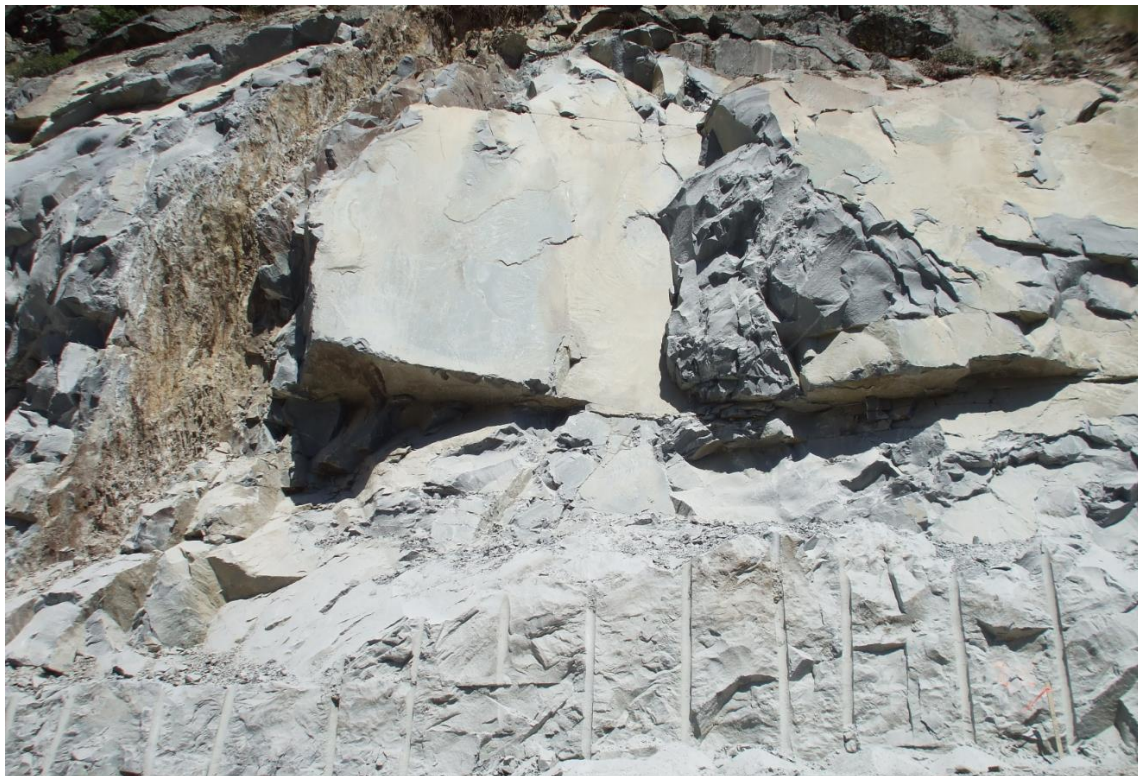
Ten Mile Rock Quarry, June 2013. The 10 mile quarry site is the source where rock slabs and boulders are collected and brought to the lower west Ten Mile Borrow area for processing. The material is used in the creek realignment area and the barrier wall platform.
