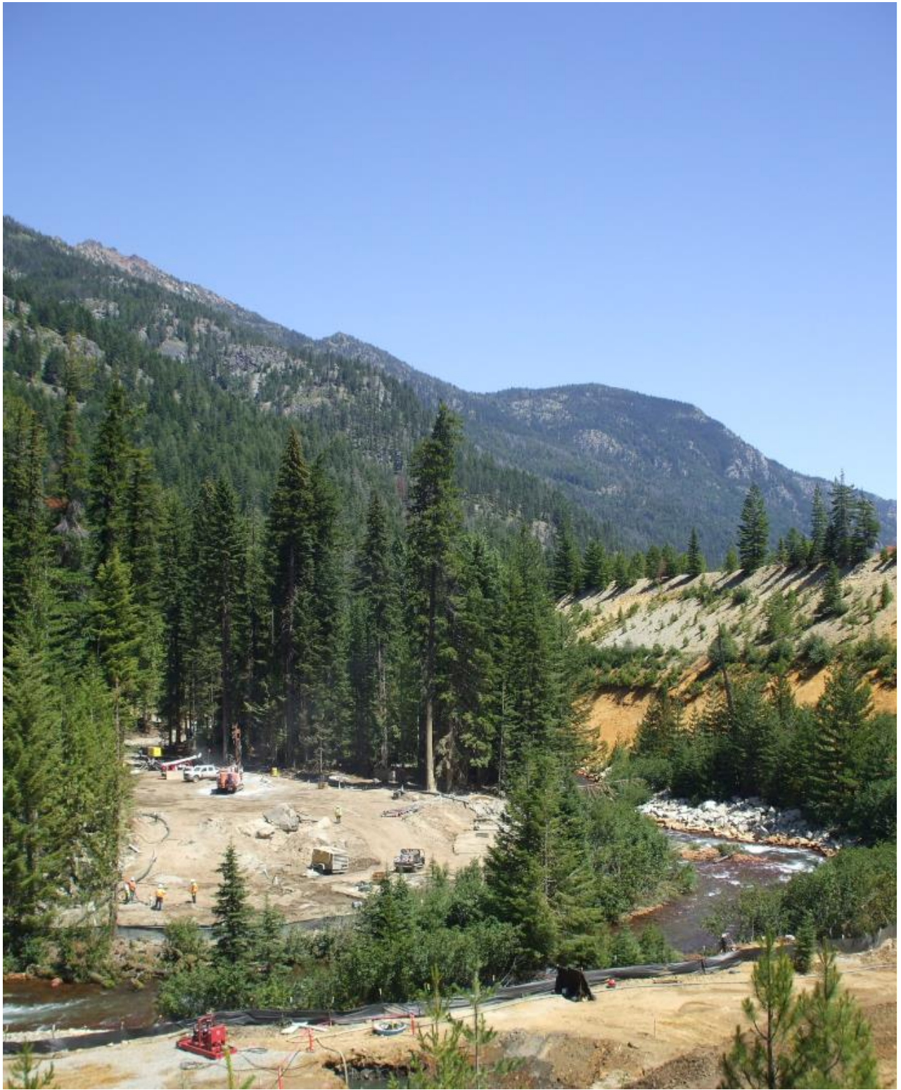
Railroad Creek alignment.
