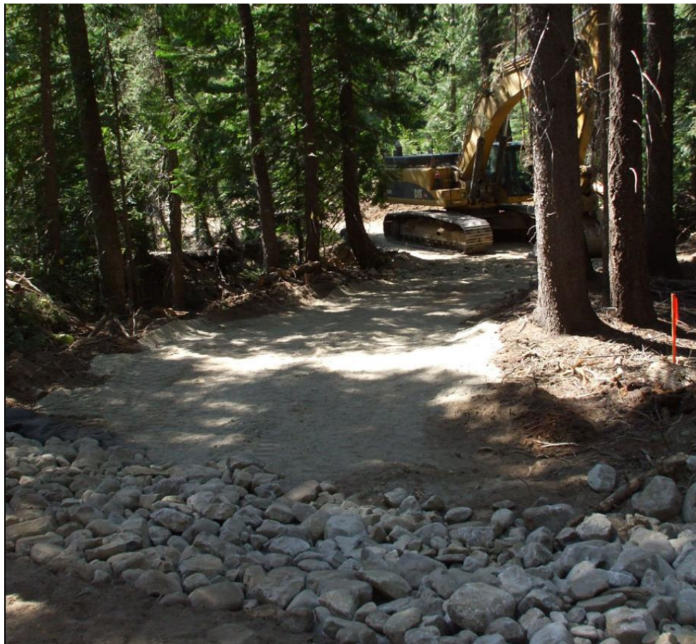
Rock Quarry investigation road.
