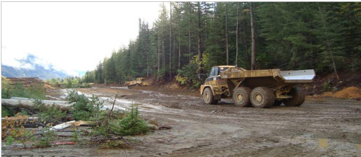
Bypass road development.
