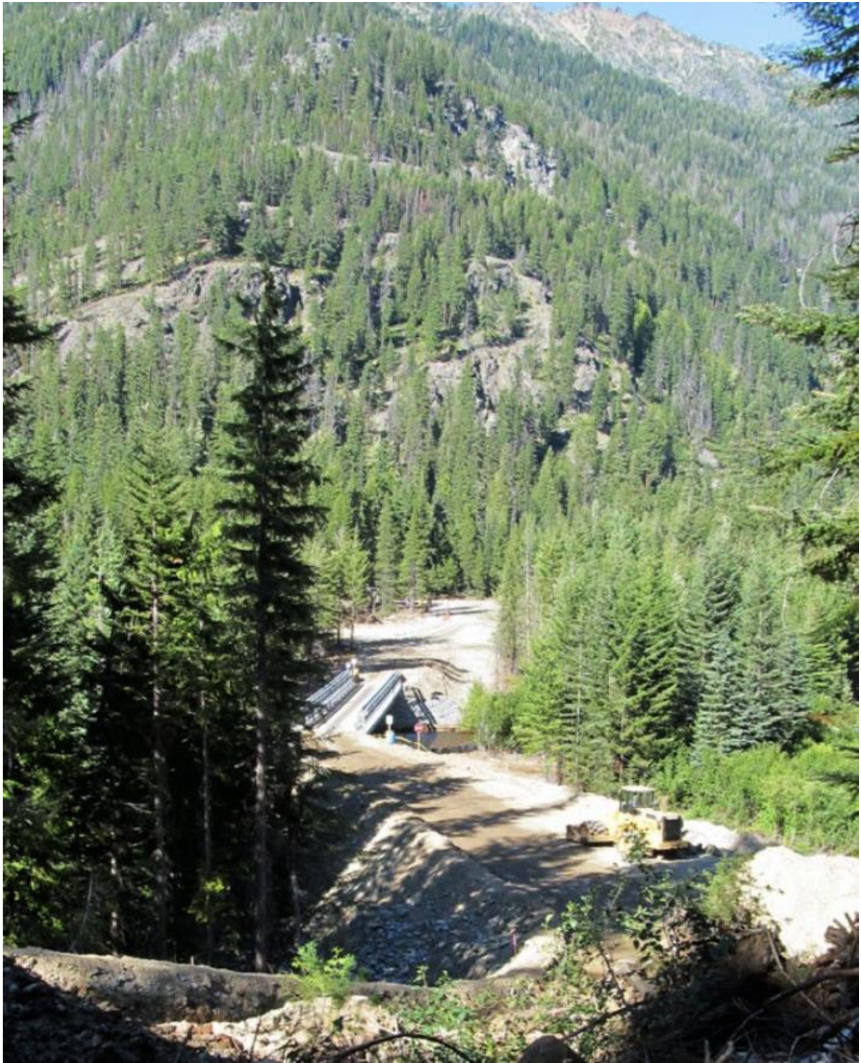
Bypass road looking towards the bypass bridge over Railroad Creek.
