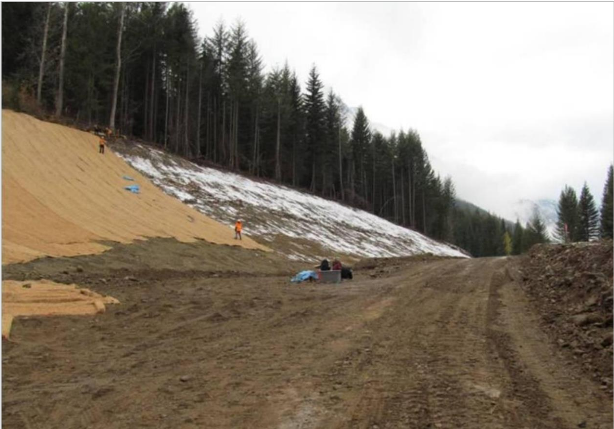
Bypass road slope erosion control blanket.
