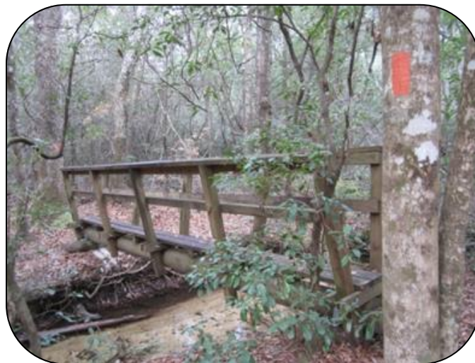
Span bridge at Eglin AFB credit: Jim Schmid
