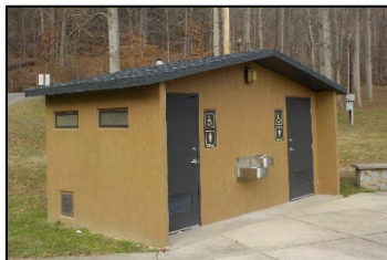
Freshly painted restroom at Lake Vesuvius Big Bend Beach
