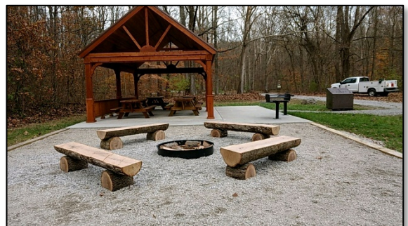
The new shelter and fire pit at Pine Hills Campground
