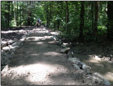
Newly constructed gravel turnpike.
