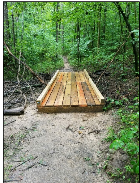
New puncheon on the Grubb Ridge trail.
