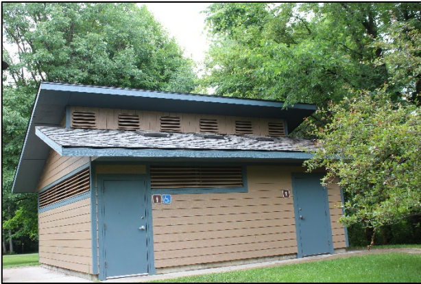
Remodeled exterior Stony Point Bathroom Building
