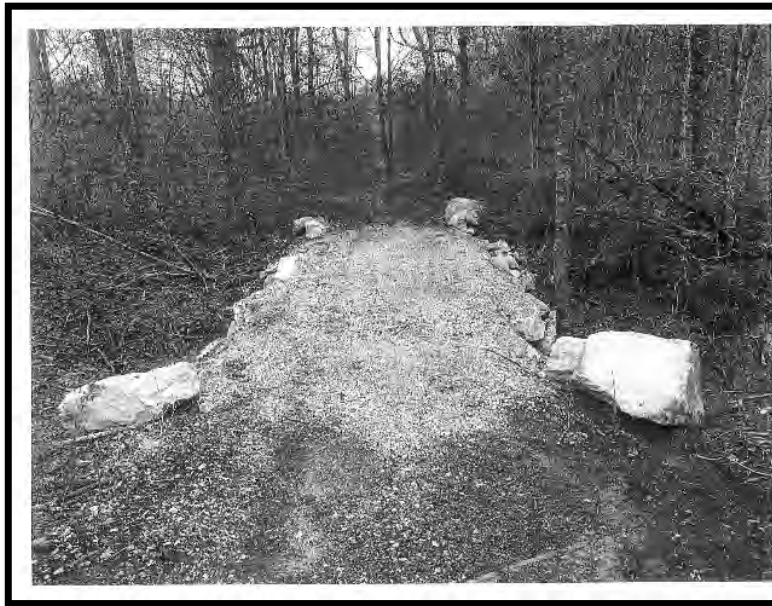
Figure 28 - Trail tread repair and culvert replacement on Hanging Rock OHV Trail
