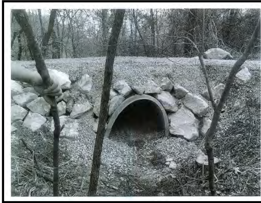
Figure 29 - Trail tread repair and culvert replacement on Hanging Rock OHV Trail
