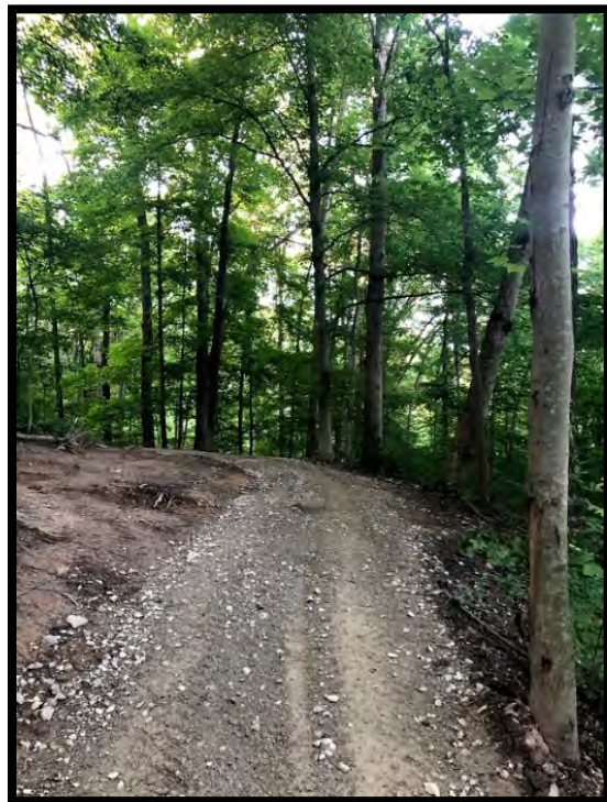
Figure 25 - Section of Dorr Run Loop Trail after maintenance
