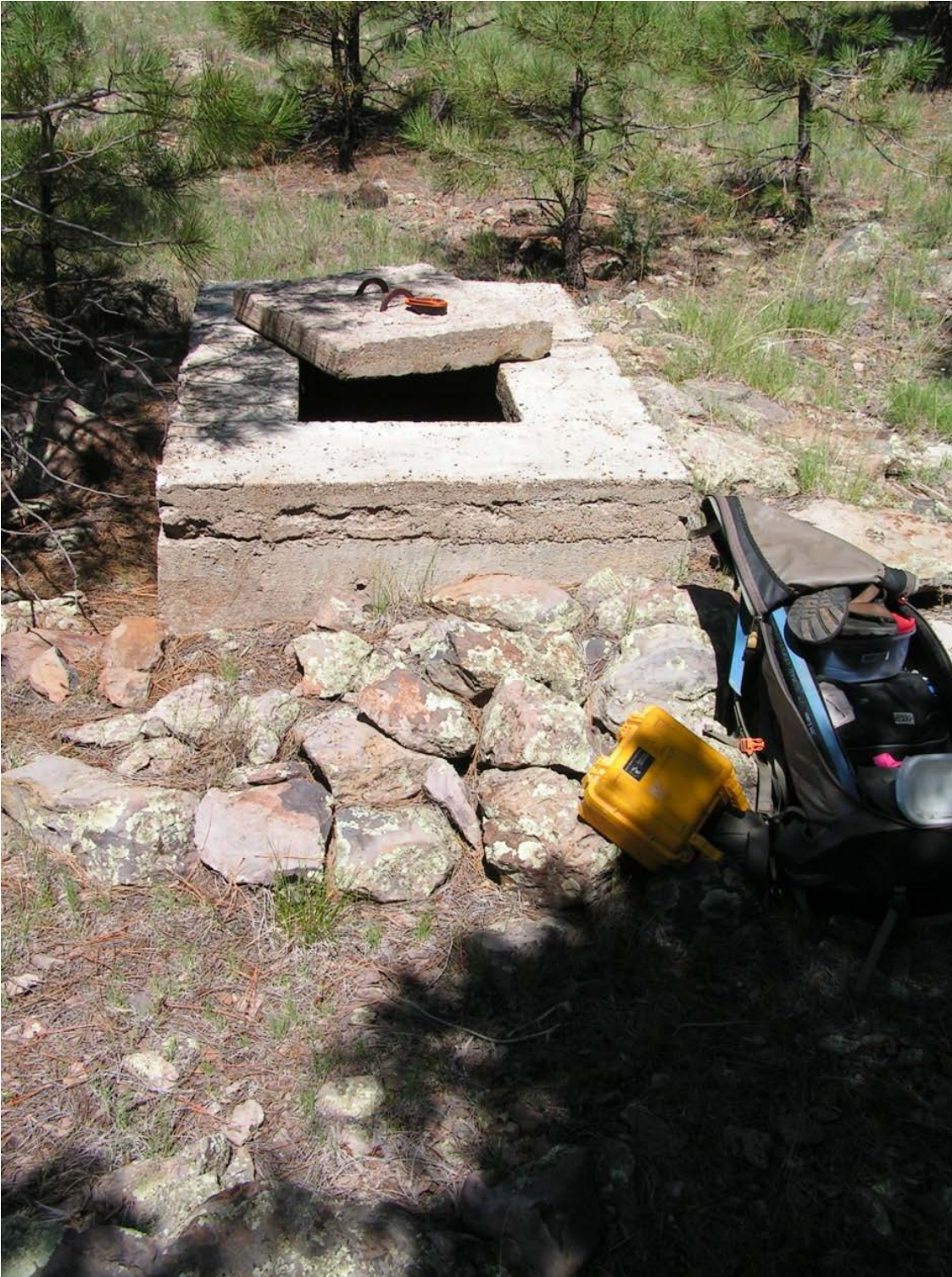
Figure 1. Photograph of Isham Spring on the Williams Ranger District, Kaibab National Forest. Note concrete spring box. This spring was dry at time of assessment in 2011. Photo courtesy of Spring Stewardship Institute (SSI).
