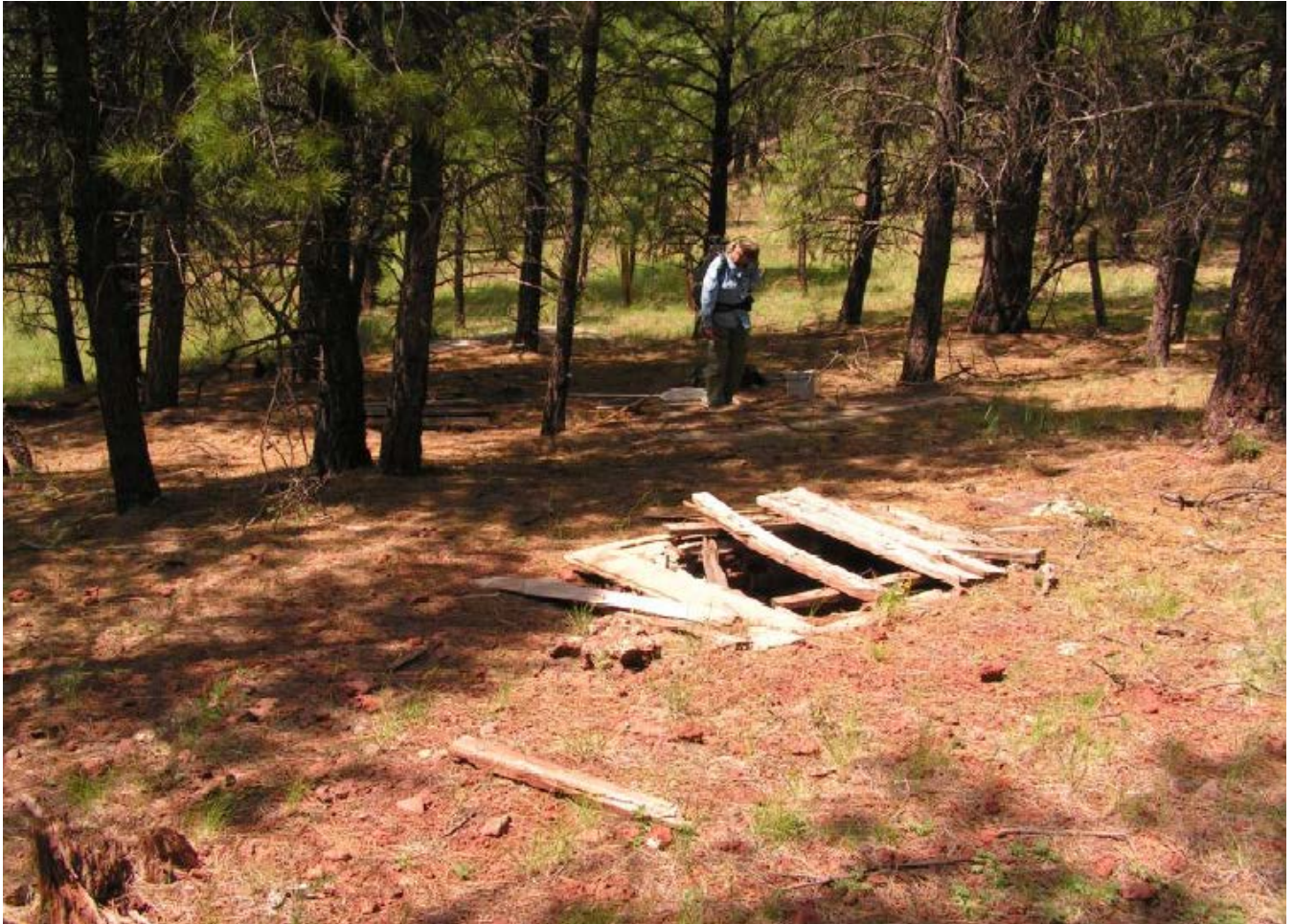
Figure 2. Photo of Lower McDermit Spring on the Williams Ranger District, Kaibab National Forest. Note dilapidated wooden infrastructure. Photo courtesy of Spring Stewardship Institute (SSI).
