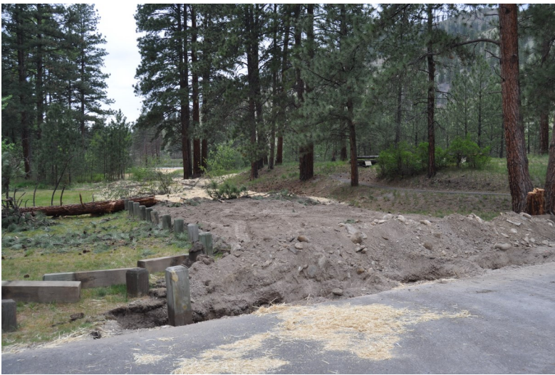
Recent road decommissioning work accomplished at Fort Fizzle.
