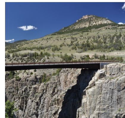
Sunlight Creek bridge, Wyoming Hwy 296. Roger Peterson, U.S. Forest Service photo
