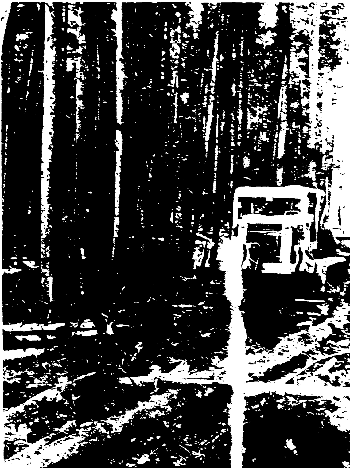
Illus. 13 Unit Piling on "Operation Pushover"
