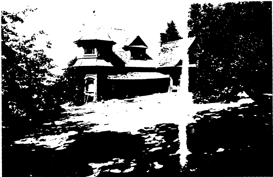
Illus. 19 Flood Damage to Home Near Ford Creek 1923
