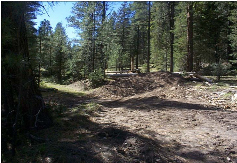
Figure 36. Slope ripping and re-contouring decommission method
