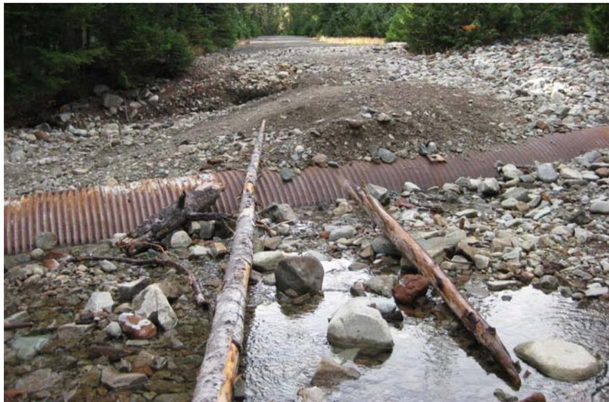
The road crossing failed when the 60” pipe filled with rock and sand being transported by the creek. This forced floodwaters over the top of the road causing the current exposed pipe condition.
