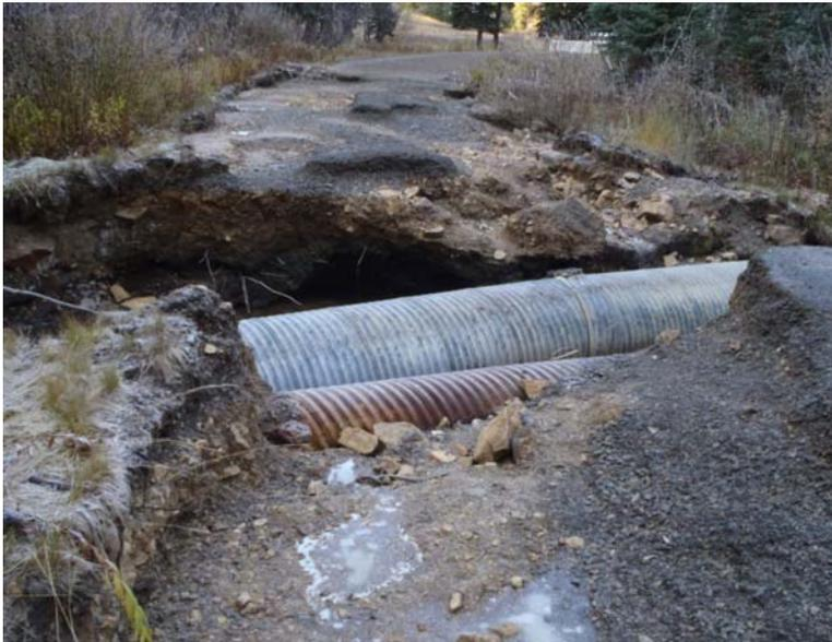
done solely by the Forest Service. At this site, the pipe culverts failed allowing floodwaters to flow over the road surface. Approximately 70 feet of road was damaged.
