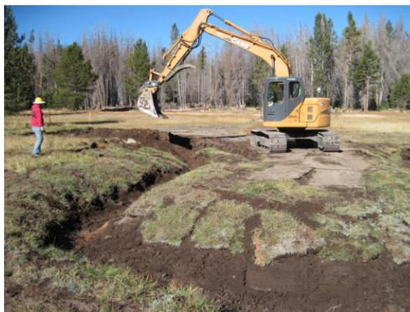
Photo 5: Cutting a new stream channel for Cold Creek in High Meadows.
