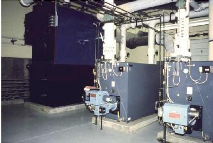
Biomass boiler (far left) with oil-fired back up boilers (center and right)
