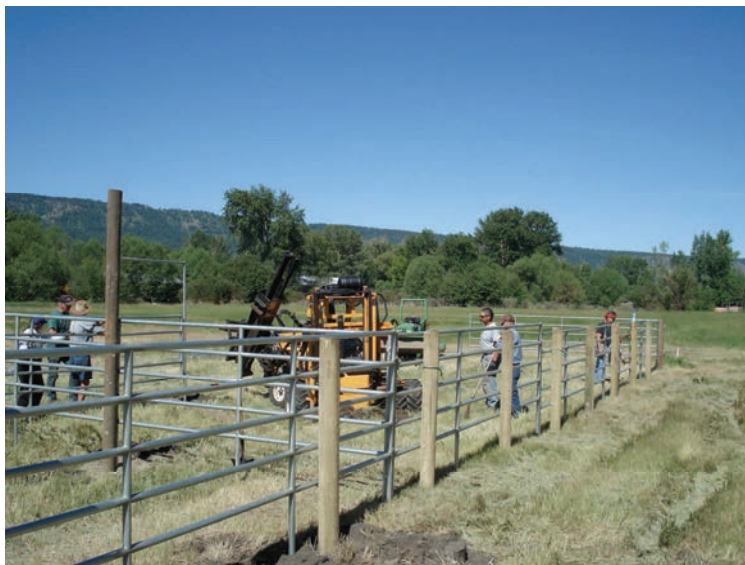
Volunteers constructing the corrals
