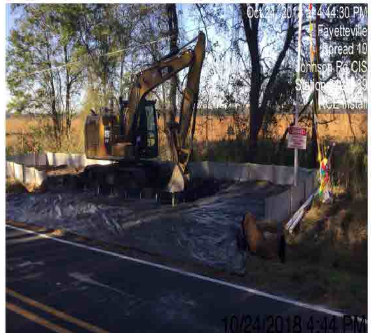
Spread 10 – Installing construction entrance to ROW
