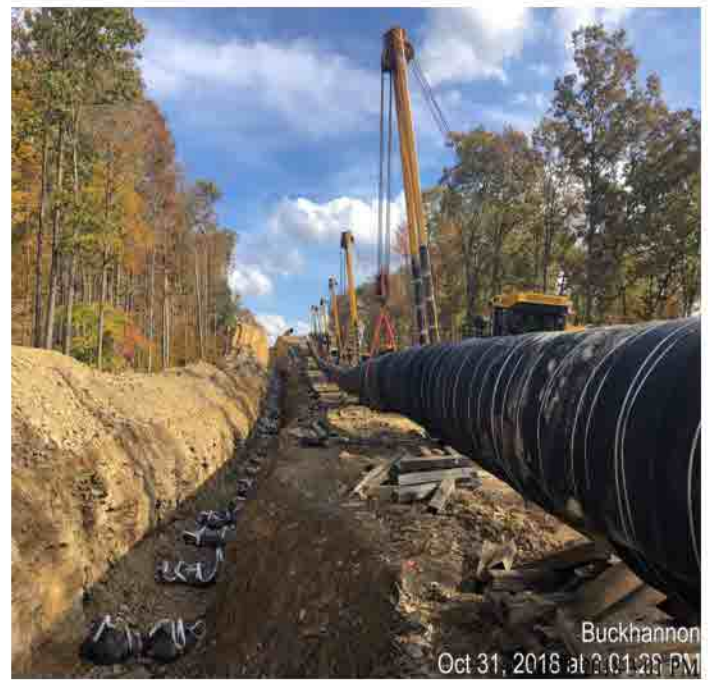
Spread 2-1 – Lowering in section of pipe
