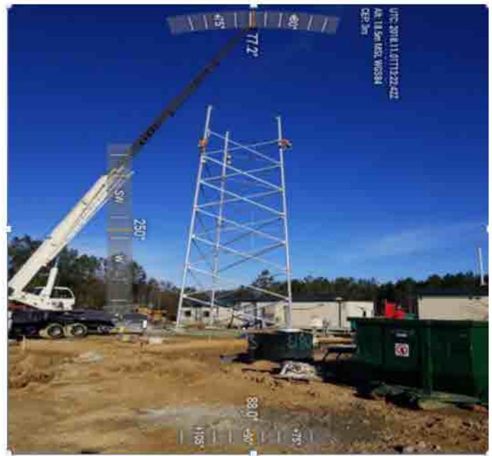
Smithfield M&R – Erecting microwave tower
