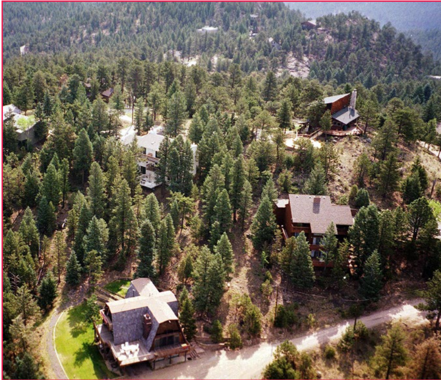
Houses in the red zone in Colorado's wildland-urban interface (WUI). Over 2 million people live in Colorado's WUI, making it more important than ever for communities to engage in wildfire risk reduction through community wildfire protection plans. Photo: Colorado State Forest Service (2015).
