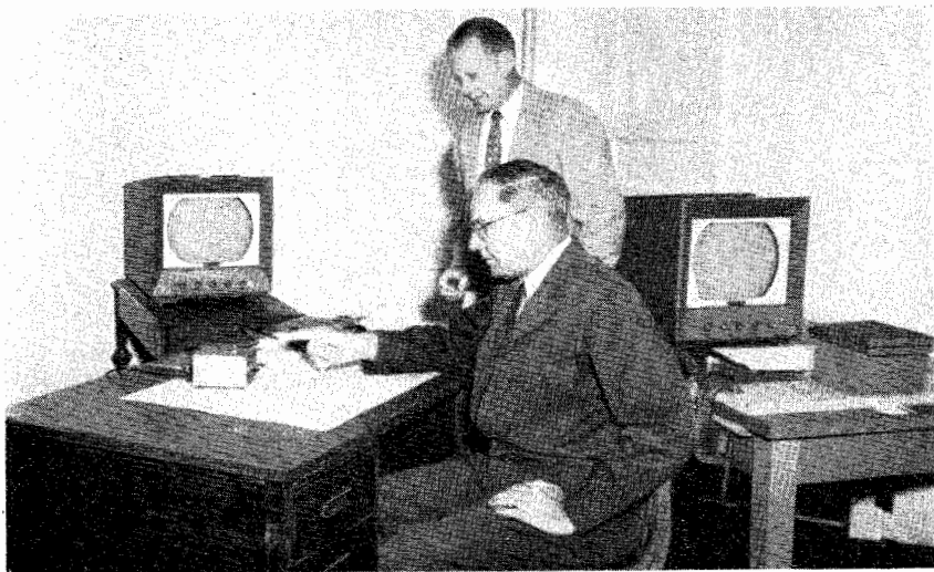
FIGURE 1.—Monitors used in viewing by TV lookout-observer and in taking pictures of scene observed; remote control unit on desk.
