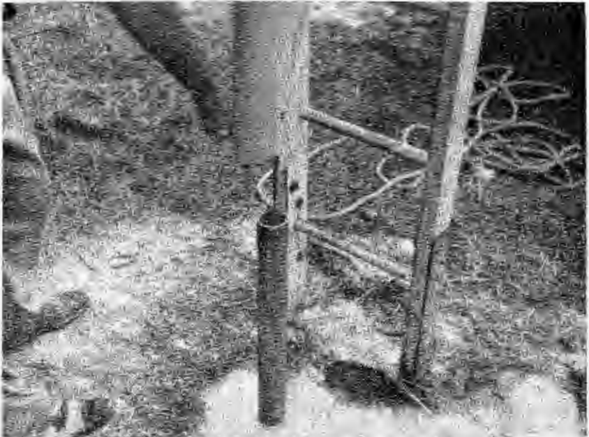
FIGURE 2.—Suction pipe and well screen placed in well ready for pumping.
