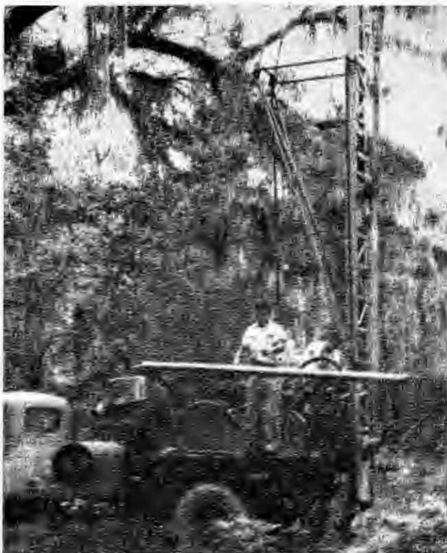
FIGURE 3.—Commercial drilling equipment in place.
