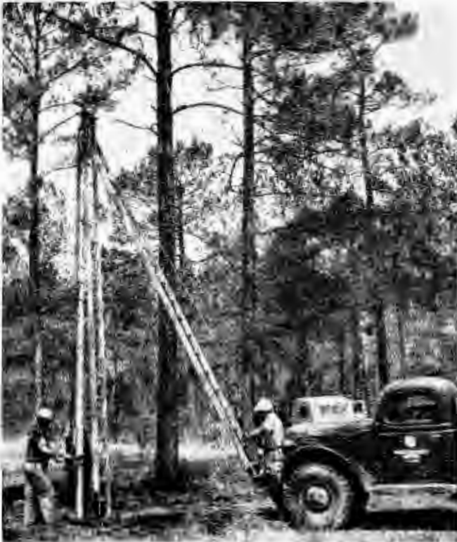
FIGURE 1.—A 4-inch casing ready to be lowered by hydraulic method. The derrick is positioned and the well casing and washing nozzle are in place ready to start pumping operation.
