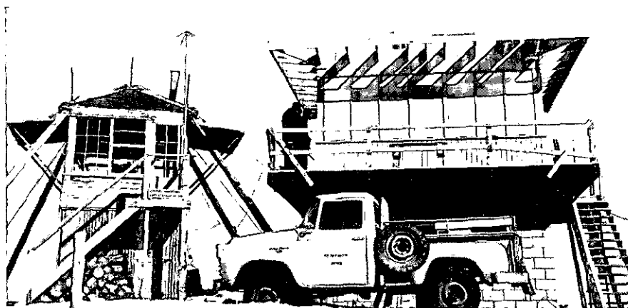
Old and new lookouts on Garnet Mountain on the Gallatin National Forest in Montana. The old lookout was erected in 1949; the new two-story flat, in 1962 (Lew Peck, 1962). 503633
