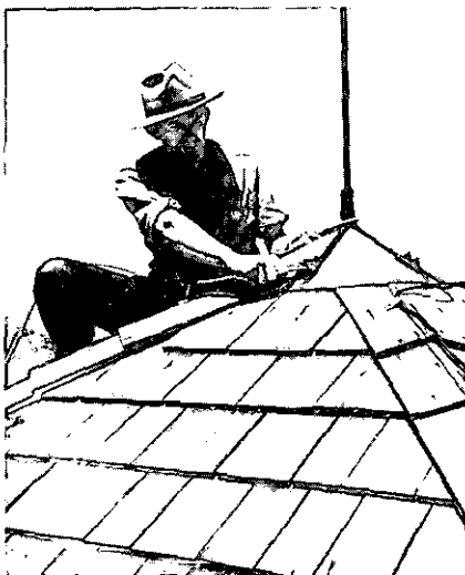
Lookout on Arapaho National Forest in Colorado tightens connections from lead-off spike to beginning of lightning protection cage (Jay Higgins, 1949). 457737
