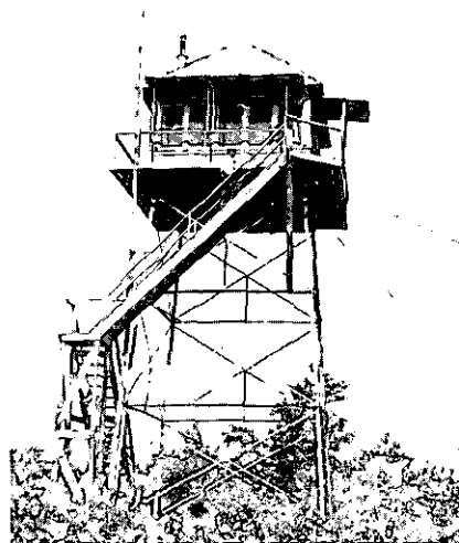
Cold Knob Fire Tower on the Allegheny National Forest in Pennsylvania (E.S. Shipp, 1926). 211642
