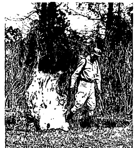
Kerosene torch used to test flammability of pasture firebreak at the Tidewater Research Center in North Carolina (W.O. Shepperd, 1950). 465050
