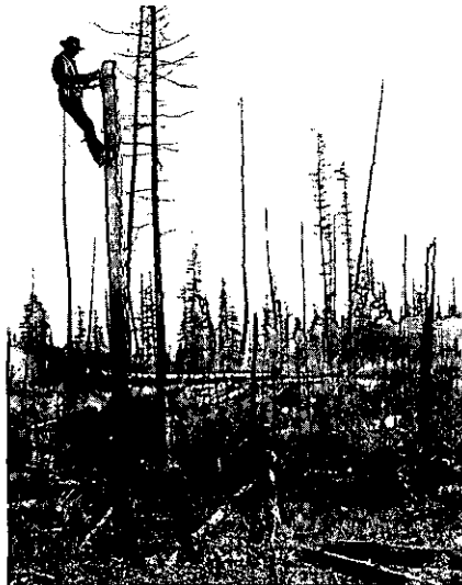
Telephone line construction through Flathead National Forest in Montana (1908). 80574
