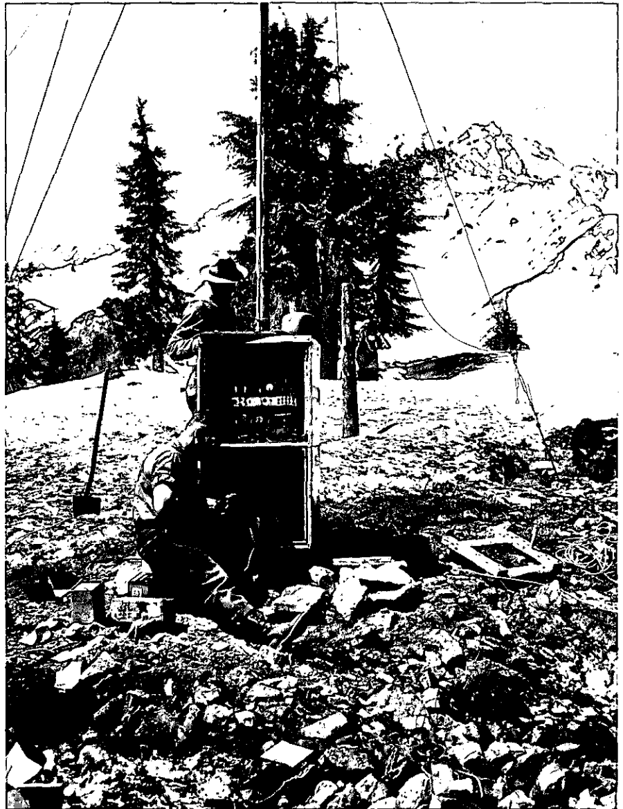
Grey Butte Radio Relay Station on Shasta National Forest in California (Fred Funke, 1941). 414468
