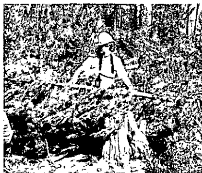
Cut seedlings and pole-sized saplings were randomly packed into the surrounding timbered area so the constructed helispot would more closely resemble a natural appearing landscape.
