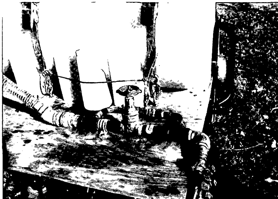
The eductor plumbed into the firefighting apparatus.
