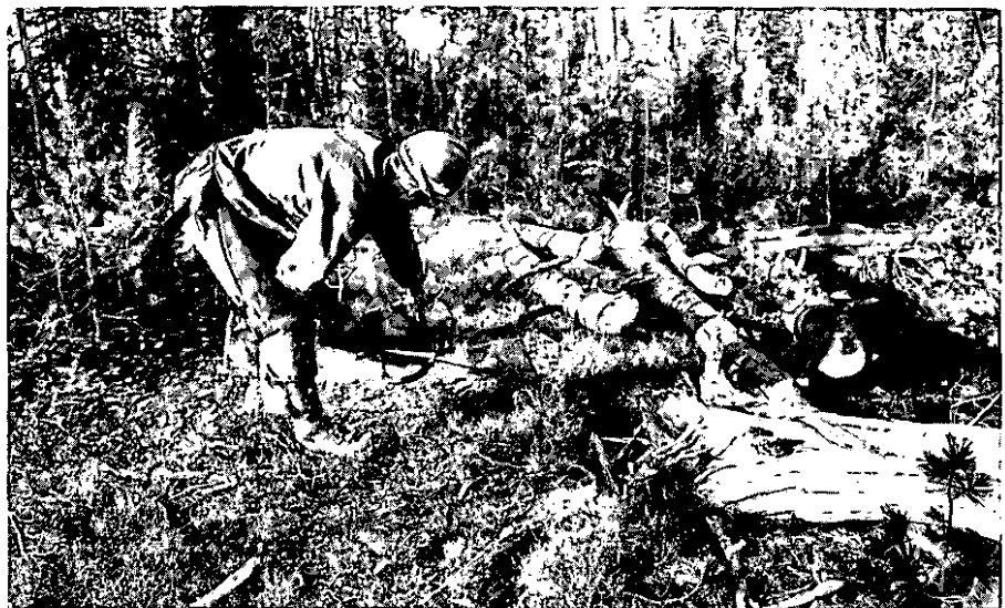
A member of the Zig Zag Interagency Hotshot Crew flush-cuts one of several stumps that resulted during helispot construction.
