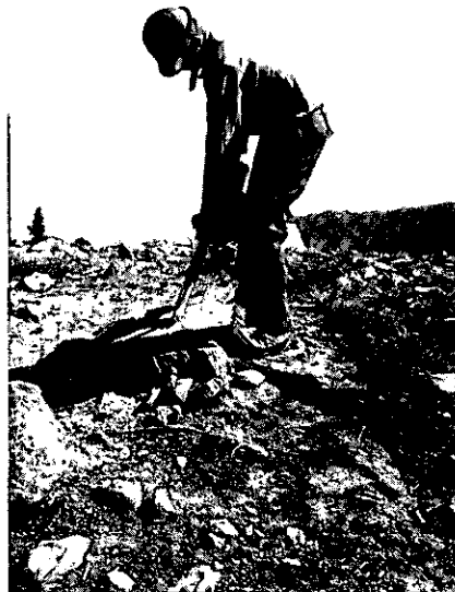
North Fork Ranger District certified blaster Don Smith makes a hole in the top of a stump (from a tree cut during helispot construction) to install explosives. Using explosives on cut faces of stumps and boles is a technique to make them look natural. Photo credits: All photos in this article are by Francis Mohr, Wallowa-Whitman National Forest.
