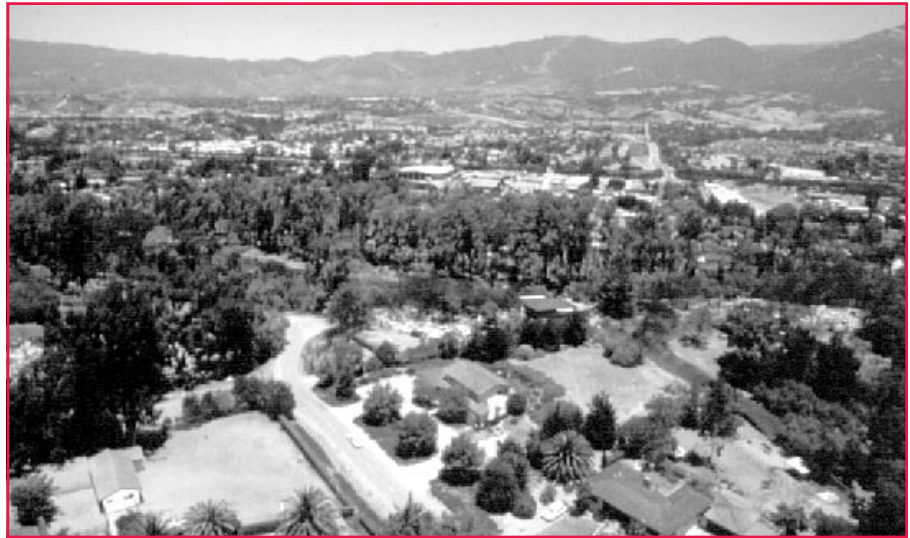
Post-burn aerial views show an area of the Los Padres National Forest in California where firefighters were able to hold the fireline and protect homes because the fuel load was relatively low in this neighborhood, e.g., there was sufficient “defensible space” around structures. Photo: USDA Forest Service, Washington, DC, 1990.
