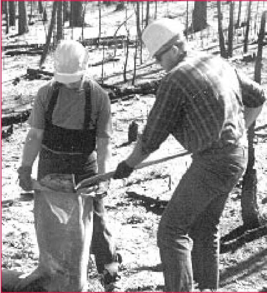
Saturdays after the fire and flood meant volunteer days in Buffalo Creek. Volunteers checked in and received safety instructions; they worked in pairs, filling gravel bags and making check dams in headwater drainages to reduce the velocity of downslope erosion. Photo: Amy Small, USDA Forest Service, Pike and San Isabel National Forests, South Platte Ranger District, Morrison, CO, 1996.
