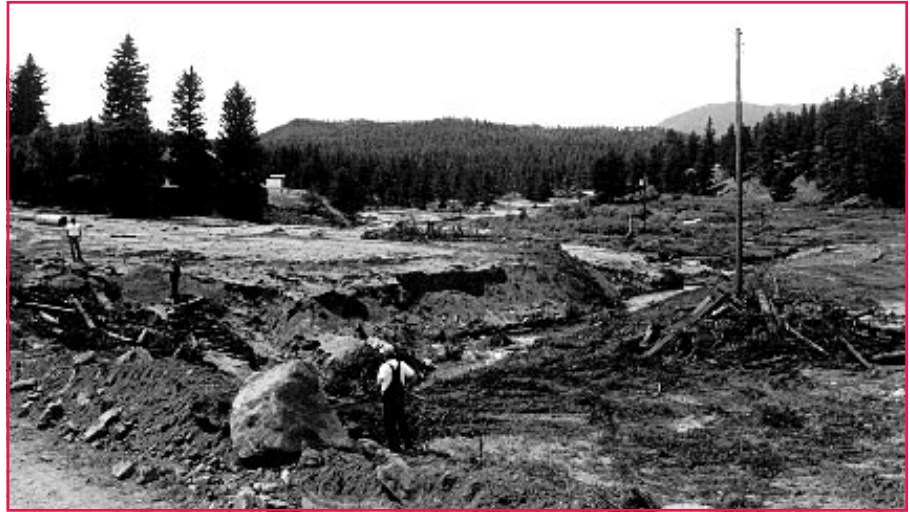
The aftermath of the flood, looking west along Buffalo Creek from what is left of County Road 126. Evidence of the earlier wildfire can be seen on the ridgetop in the distance. Over 8 feet (2.4 m) of sediment aggraded in the drainage and in and around the town. Photo: Dave Grove, USDA Forest Service, Pike and San Isabel National Forests, South Platte Ranger District, Morrison, CO, 1996.
