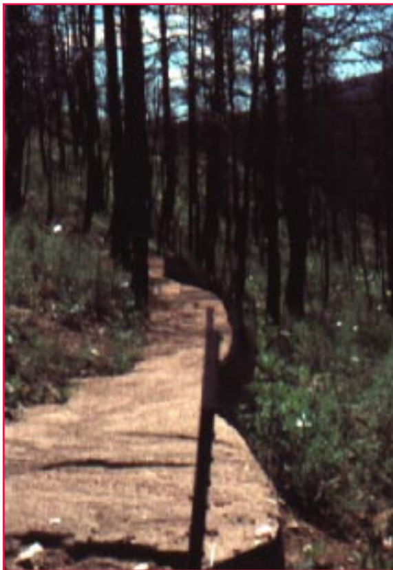
Figure 2 —Silt fence installed in Black Tiger Gulch, CO, after a severe fire in 1989. Notice that accumulated sediment is much heavier in July 1990 (left) than in May 1997 (right). Because most erosion occurs during the first year after a fire, water bars are most effective for postfire erosion control when installed shortly after a fire. Photos: Courtesy of John Winchester, Boulder, CO, ©1990 and ©1997.
