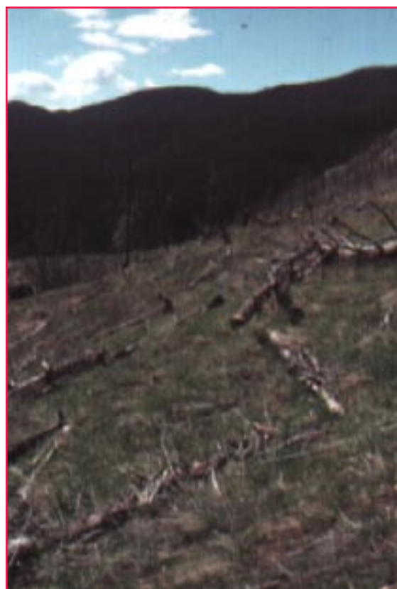
Figure 1 —Ineffectively installed water bars in Black Tiger Gulch, CO. After a severe fire in 1989, trees were felled cross-slope for erosion control. Notice that between May 1990 (left) and May 1997 (right), no sediment accumulated behind the water bars. Inadequate installation permitted water flowing downhill to form rills under the trunks, rendering them useless as water bars. Photos: Courtesy of John Winchester, Boulder, CO, ©1990 and ©1997.
