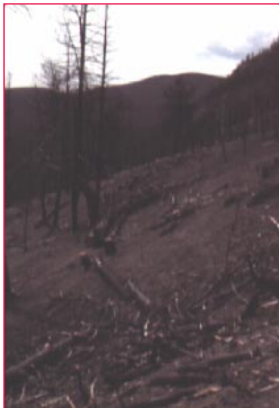
Figure 1 —Ineffectively installed water bars in Black Tiger Gulch, CO. After a severe fire in 1989, trees were felled cross-slope for erosion control. Notice that between May 1990 (left) and May 1997 (right), no sediment accumulated behind the water bars. Inadequate installation permitted water flowing downhill to form rills under the trunks, rendering them useless as water bars. Photos: Courtesy of John Winchester, Boulder, CO, ©1990 and ©1997.
