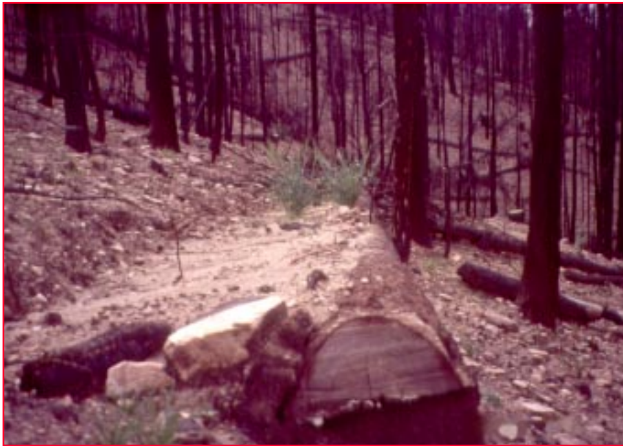
Log erosion barrier installed on a slope following the Viveash Fire. Photo: Wayne Robbie, USDA Forest Service, Albuquerque, NM, 2001.
