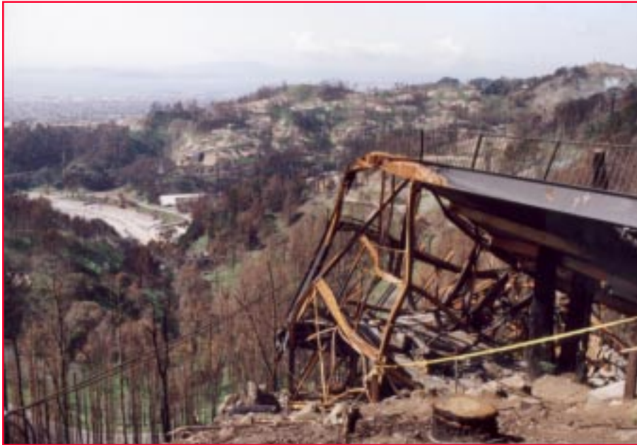
Neighborhood devastated by the 1991 Oakland Hills Fire, about 6 months after the event. Buckling of a steel platform (above), once part of a hillside home, indicates the intensity of the firestorm, which destroyed some 2,900 structures and took 25 lives in residential parts of Oakland and Berkeley, CA. Logs and snags frame the chimney of a surviving home (below), remnants of the thick intermix vegetation that fueled the flames. Photos: Hutch Brown, USDA Forest Service, Washington, DC, 1992.
