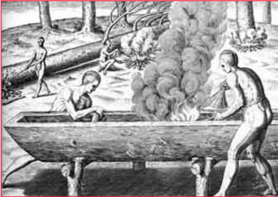
“The manner of making their boates [sic],” from a drawing in about 1585 by John White near the ill-fated Roanoke colony in what is now coastal North Carolina. Coastal tribes made canoes by using fire to hollow out large trees (foreground). Fire also gave them the technology they needed to fell large trees (background, upper right) and buck the boles (upper left). They would have used the technology not only for boatmaking, but also for agricultural clearing and acquiring timber for village palisades and buildings.
