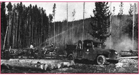
**Figure 2**—*A jeep tanker being tested prior to the broadcast burning of an area of lodgepole pine slash on the Deerlodge National Forest in Montana. Photo: USDA Forest Service.*
