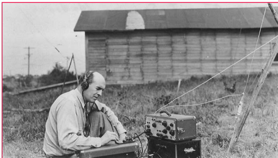
Forest Service radio pioneer Dwight Beatty operating his SP-1930 (Semi-Portable) Morse Code transceiver. Eight of these units were produced for fireline communications and testing. Photo: Forest Service, James Allen collection, Los Altos, CA.
