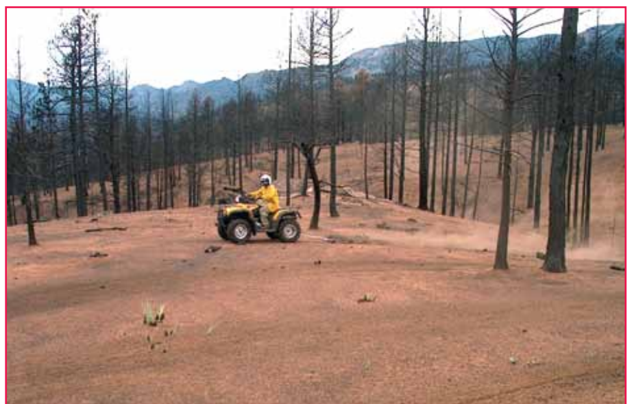
Figure 2—The scarify-and-seed treatment was implemented on 13,200 acres (4,340 hectares) of moderately to severely burned Forest Service land in the months following the Hayman Fire. Scarification was done in rows either by all-terrain vehicles pulling harrows (as shown in the photo) or by hand with McLeods. Barley and triticale seeds were spread on the scarified areas. Photo: Pete Robichaud.
