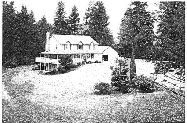
Firewise houses create a landscape that is lean, clean, and green for at least 30' around the house. Fire resistant material on the roof and walls adds protection from a wildfire. For more information, check www.firewise.org on the internet. Photo courtesy of WA State Department of Natural Resources
