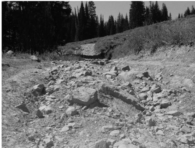
**Figure 1.1 Large, angular rock in the Logan Peak Road (20042)**
