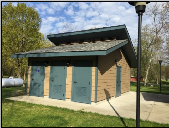
New and improved Stony Point Shower Building
