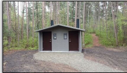
New vault toilet at Norway Beach Recreation Area.
