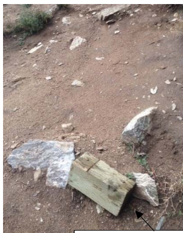
Belay footing station at Tick Wall Route Ticktastic. 1' long treated 4"x4" set with 2 rebar pieces.
