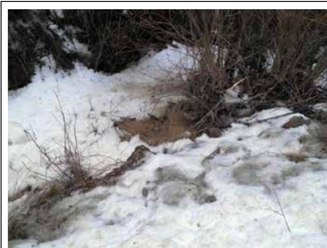
**Photo 13 – Outlet of FSR 428 Ditch Relief Culvert Carrying Water and Sediment into Ambrose Creek, February 2015**
