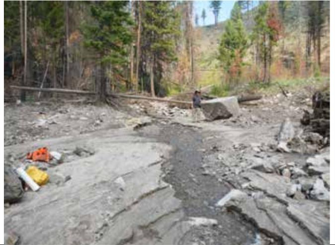
**Photo 6 - Forest Road 468 Crossing of Scimitar Creek after the Debris Flows. The 2013 Fish Culvert is Buried near the Large Boulder in the Photo, August 2014**
