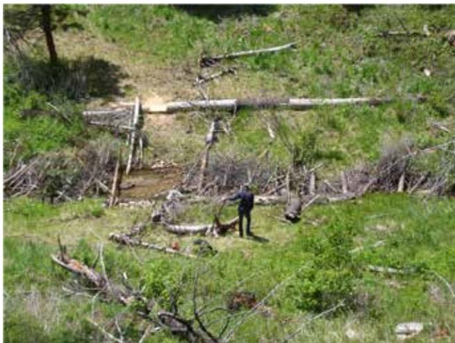
**Photo 1 - Slash Placement on a Recontoured Road 13304 Stream Crossing, June 2009**
