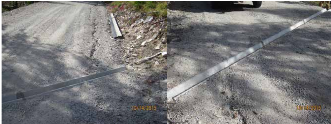
Photos 5 – Concrete Water Bar Installation Lost Trail Ski Area NFSR 5734
