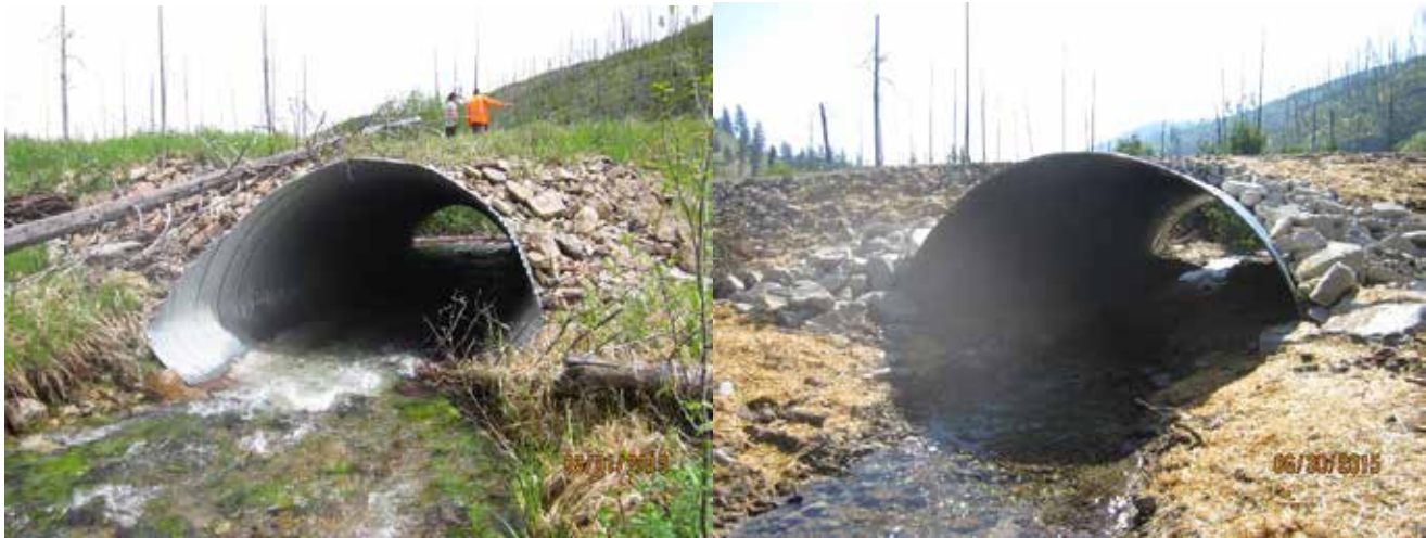
Photos 1 - Little Blue Joint Culvert Repair before and after Photos
