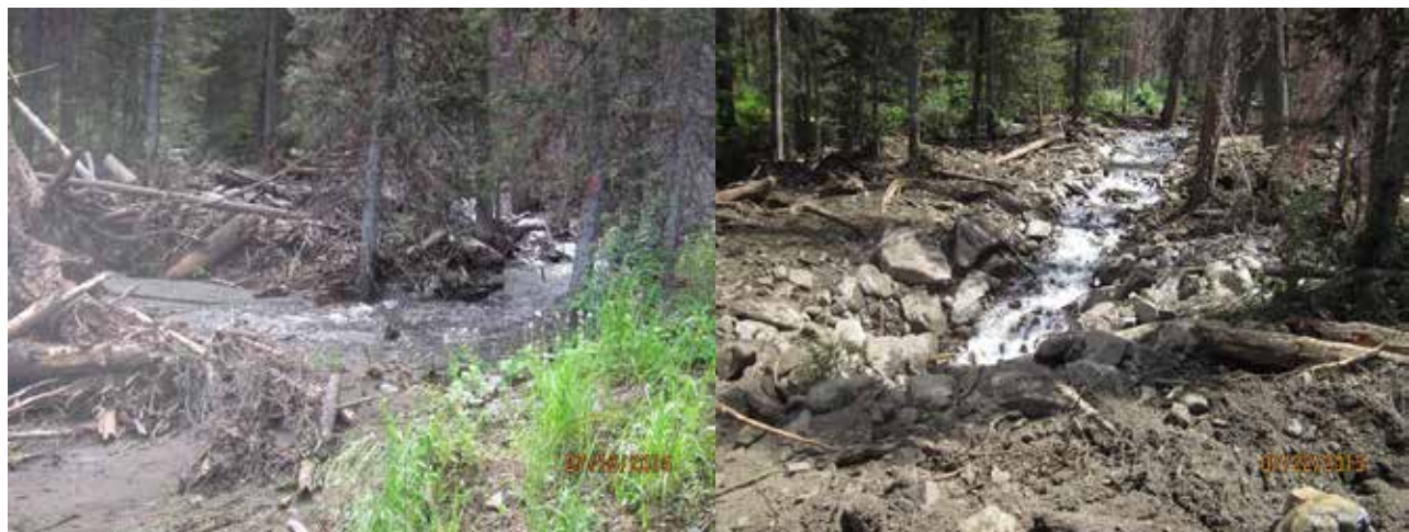
Photos 2 - Johnson Creek before and after Photos Taken from the Edge of NFSR 91
