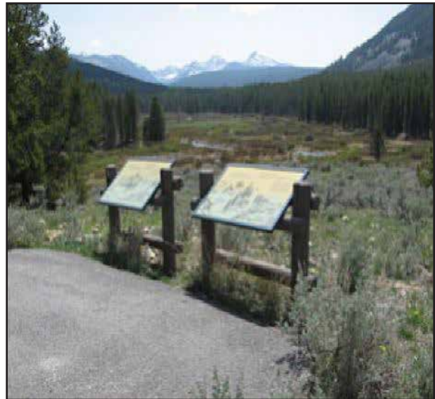
Examples of “legless” aluminum frames mounted onto a rounded timber structure (above: Beaverhead-Deerlodge NF, MT; left: Gallatin NF, MT)
