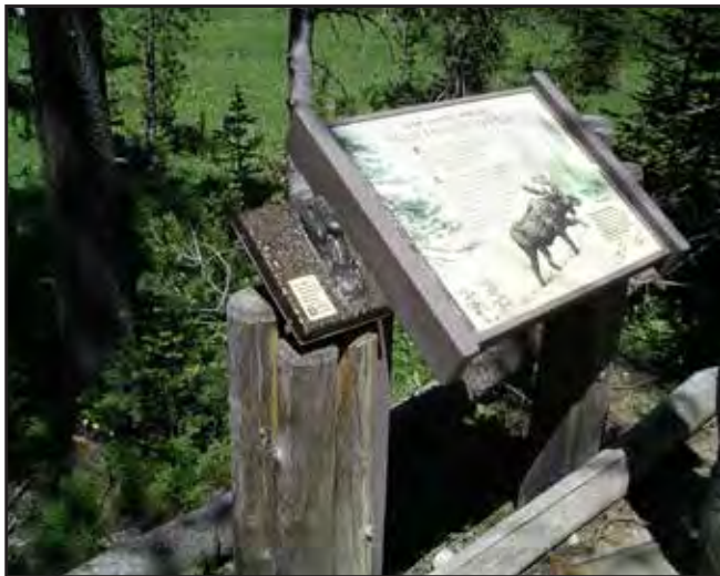
Examples of “legless” aluminum frames mounted onto a rounded timber structure (above: Beaverhead-Deerlodge NF, MT; left: Gallatin NF, MT)
