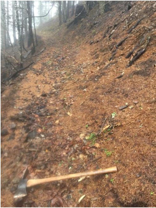
Figure 3 Moderate sloughing along sections of trail
