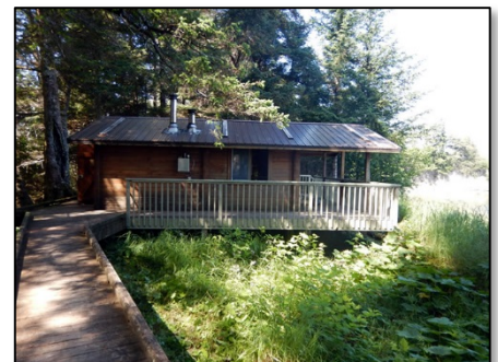
Green Island Cabin with newly stained deck railing
