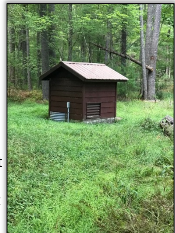
Better roof at lift station pump house
