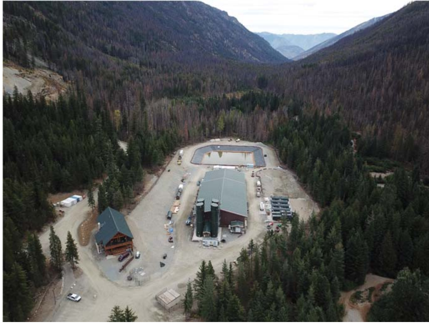
Figure 12. Water Treatment Plant at the Holden Mine Remediation Site.
