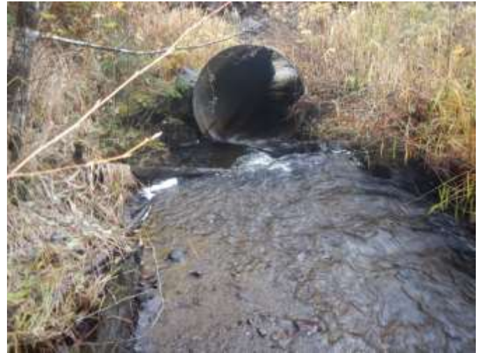
Steelhead Creek RD 2000440 MP 0.130 pre-replacement
