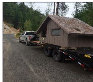
Transporting and installing the vault toilet at the Beth Lake Campground
