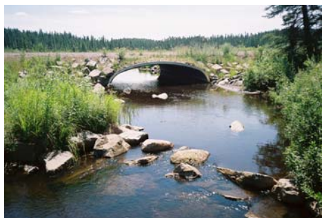
Stream crossing restoration project
