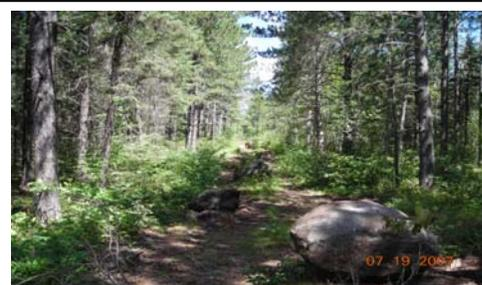
Figure 12. 2007. Nira Project. Rock placement and loosened soil along road to prevent motorized travel
