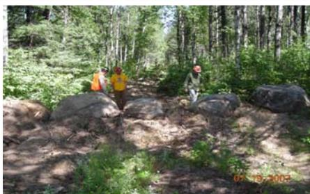
Figure 11. 2007. Nira Project. Rock placement at road entrance to prevent motorized travel
