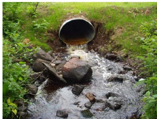
Photo 2. Existing culvert identified as a fish passage barrier during road/stream crossing surveys
