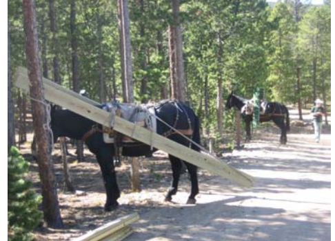
Above: The Regional pack string is loaded with bridge materials.
