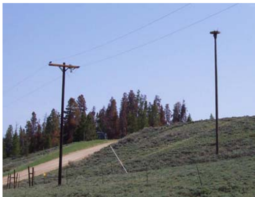
Above: New Bussey Hill Platform next to distribution pole
