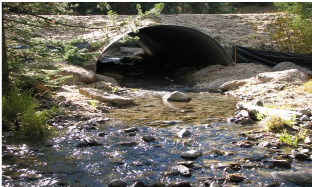
**Photo 2. Soap Creek stream simulation culvert (14' x 10' buried arch pipe) after replacement.**
