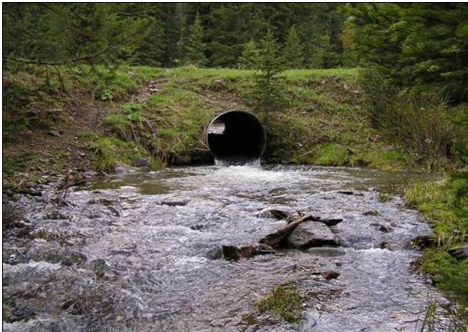
**Photo 1. Soap Creek culvert (48” diameter CMP) with perched outlet previous to replacement.**
