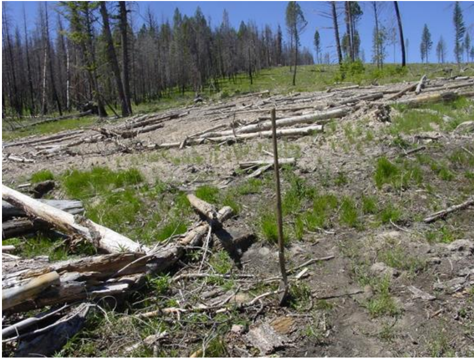
Figure 1 - Temporary Road constructed in 2009 and obliterated in 2010. Shovel is in the former temporary road bed.
