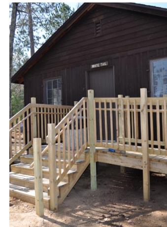
New stairs and ramps to every cabin.
