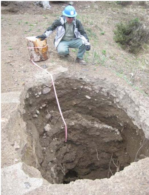
Sulphur Ranger District staff work to assess damage caused by a sinkhole on Stillwater Pass Road. An old wooden culvert beneath the road had failed during spring runoff.
